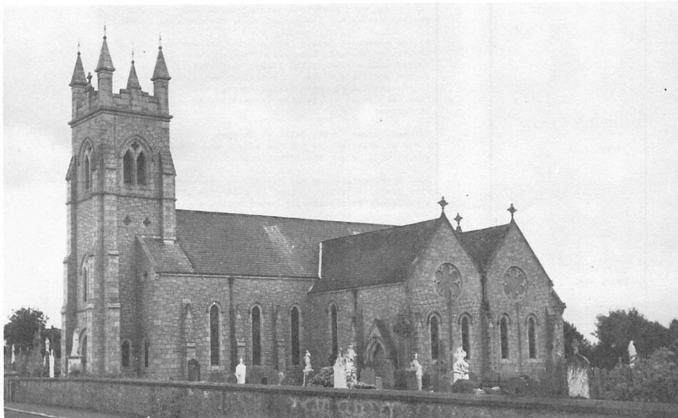
St. Colman's Roman Catholic church (Kilkeel No. 34)
